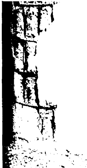
Figure 4.4: Column Corrosion Resulting for Splashing Adjacent to Roadway [West et al, 1999]
