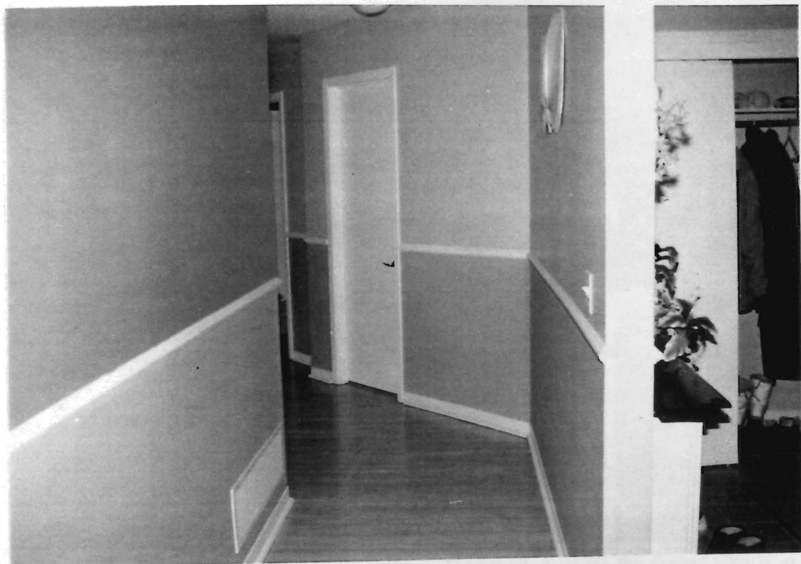
AFTER: Hallway; wide enough for wheelchair accessibility, and moulding is provided for protection against the wall from the wheelchair, but also as a guide for the blind.
