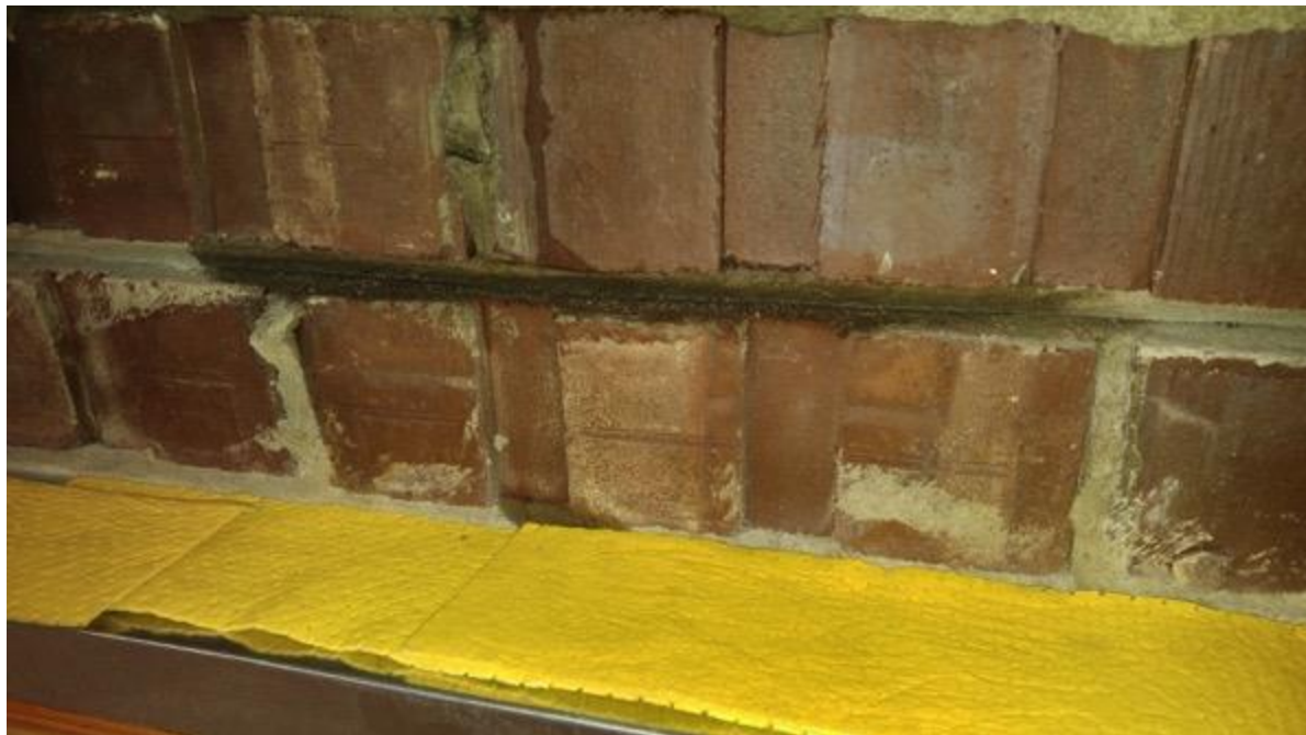
Figure 57 – Photograph showing water accumulating on a raked mortar joint, outside the test area.
