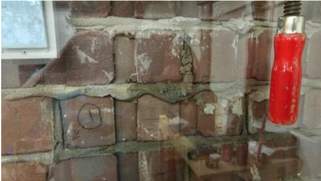
Figure 58 – Photograph showing moisture accumulation on mortar droppings.
