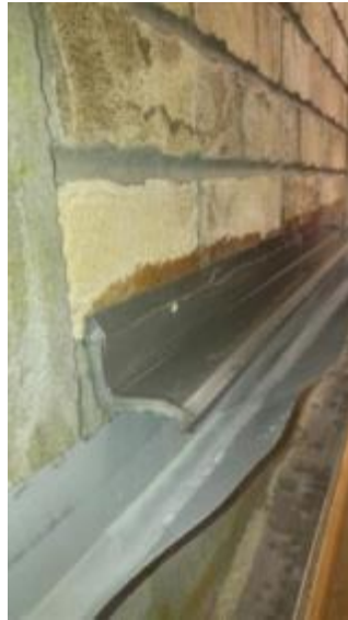
Figure 10 – Flashing and trough showing drainage path of deflected water
