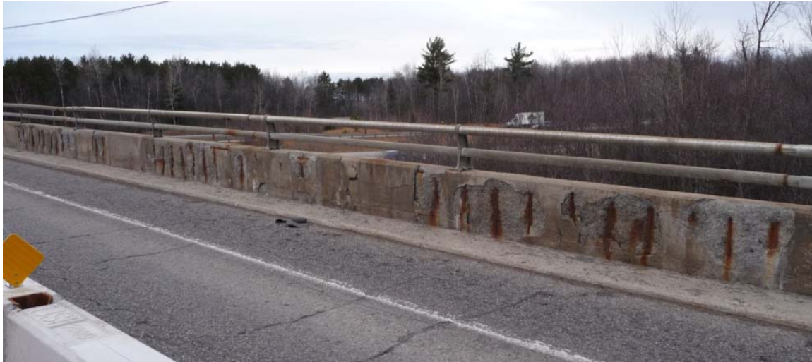
Fig. 1.1 Corrosion-induced degradation of steel-reinforced bridge barrier wall
