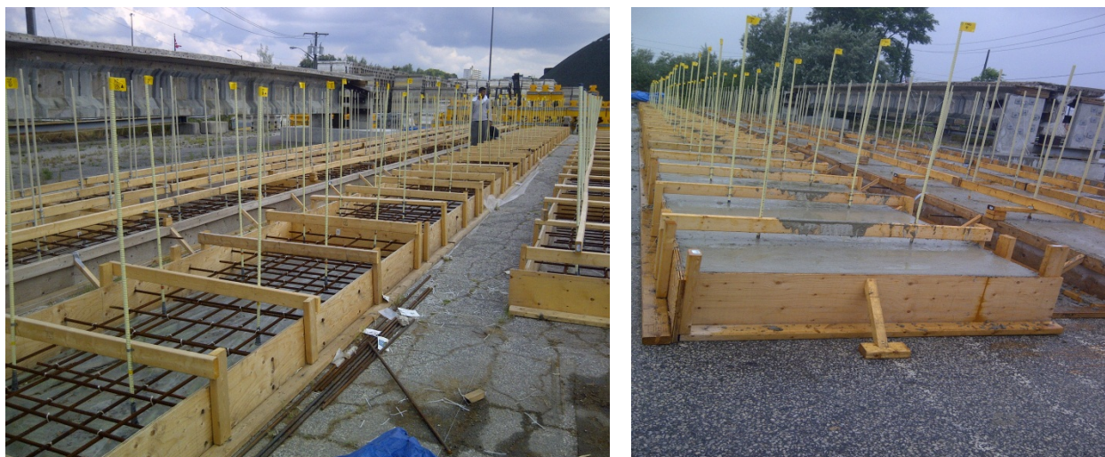
Fig. 3.2 Views of the formwork for casting concrete slabs with embedded GFRP bars
