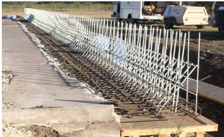
Fig. 4.3 View of reinforcement in the constructed PL-3 barrier
