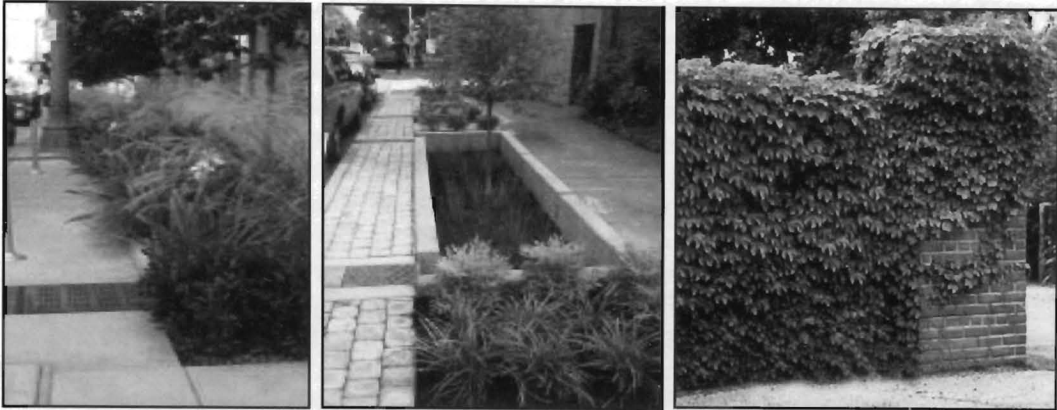
Figure 33 and 34 and 35. Laneway Landscaping Techniques – Infiltration Planter, Flow-through Planter, and 'Green Wall'.
