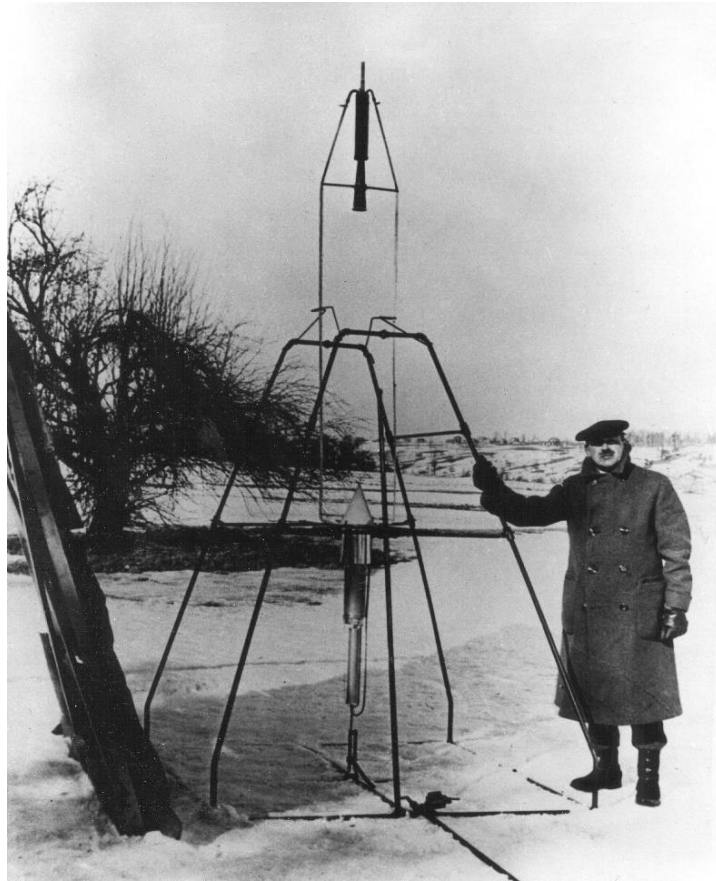
Figure 1: Robert Goddard next to the First Modern Liquid-Propellant Rocket. Courtesy of NASA.
