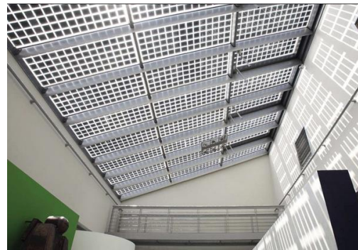
Figure 10: BIPV technology for glazing, (Google Images)
