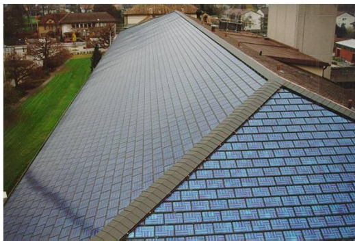
Figure 9: BIPV technology for shingles, (Lumen Solar LLC News, 2010)
