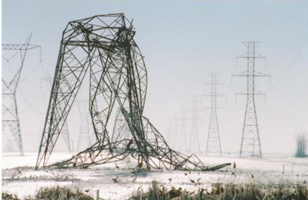
Figure 2: Collapsed high voltage transmission towers. Hydro Quebec/via Google images
