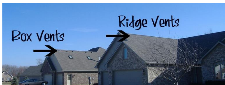
Figure 29: Ridge Roof Vents (Google Images)
