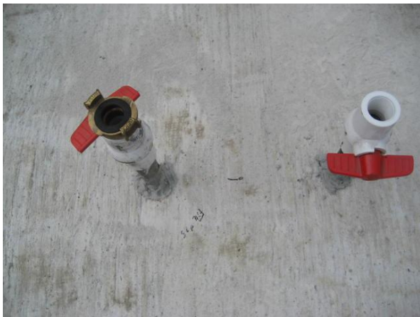
Fig. 4.73 Closing pre-drilled hole (right), tight-connection to drilled hole for grouting (left)
