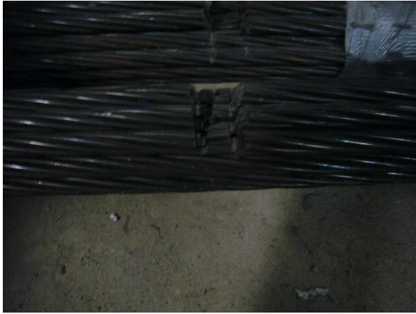
Fig. 3.5 View of the prestressing cable showing a U-shape Notch
