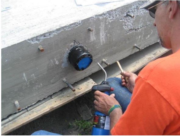
Fig. 4.68 Sealing the tendon duct from ends to prevent air leakage
