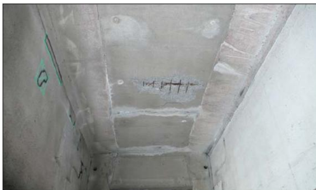
Fig. 2.42 Underside location of detected fracture (Adapted from Fallis et al., 2008)
