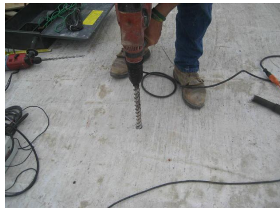
Fig. 4.71 Making larger diameter hole to the void using 25 mm diameter drill bit
