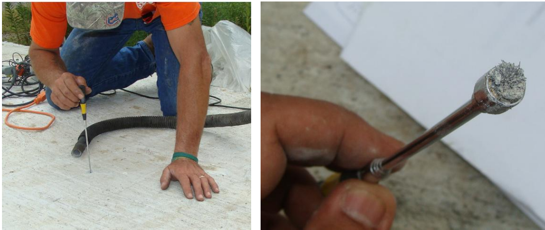
Fig. 4.76a Views of the stick with magnetic base to detect the presence of the prestressing cable at bottom of the drilled hole
