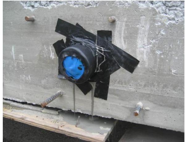
Fig. 4.76 Grout-leakage showing insufficient sealing of the tendon ends
