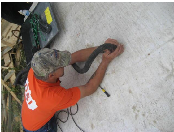
Fig. 4.70 Vacuuming out the crunched concrete from the hole
