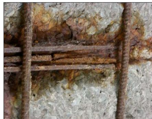
Fig. 2.43 Close-up location of detected fracture (Fallis et al., 2008)
