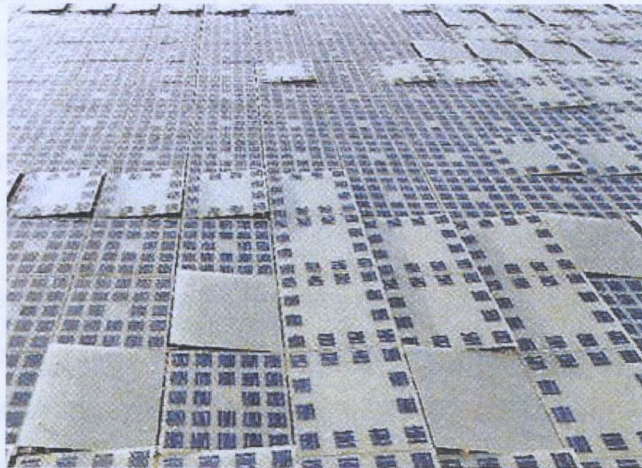
Figure 1. The Greenpix, facade integrated with photovoltaic cells and LED lighting system.
