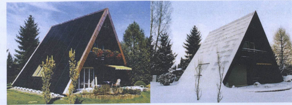
Figure 4. A vacation house in Ferienhaus Bartholoma-Park, the roof is a completely integrated photovoltaic system.
