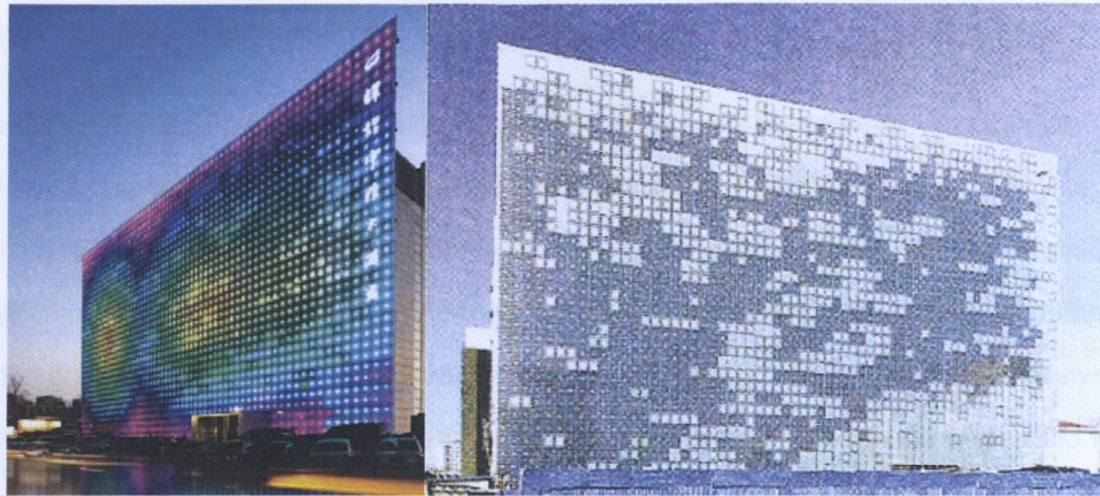
Figure 24. The Greenpix, facade integrated with photovoltaic cells and LED lighting system.
