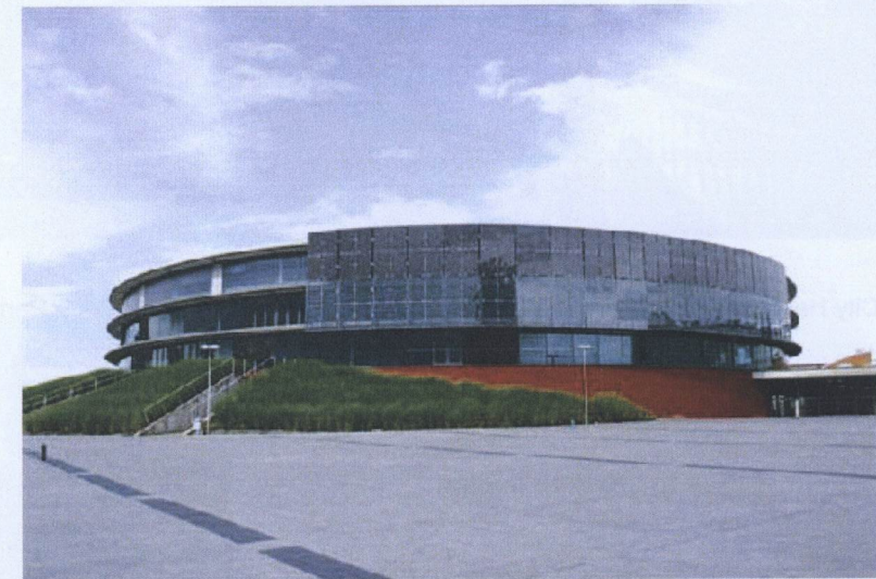
Figure 16. Oldenburg stadium EWE-Arena, cylinder shaped facade integrated with movable photovoltaic panels.
