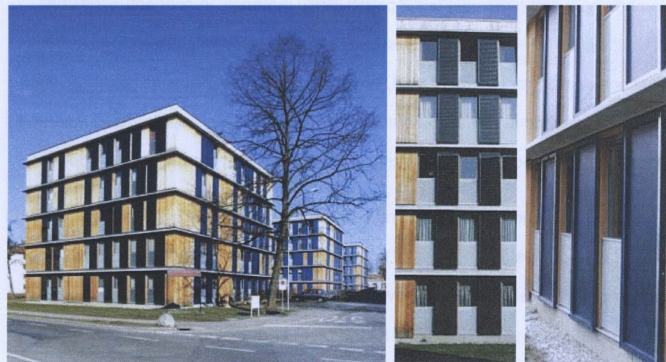
Figure 35. Spinnereistrasse in Austria: façade integrated with thin film photovoltaic panels.
