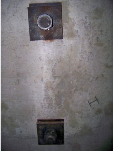
(a) Fixation of Distribution RC to Rigid wall
