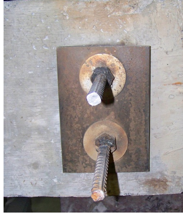
Figure 3.7: Rebars fixed to the RC beam by welding a nut
