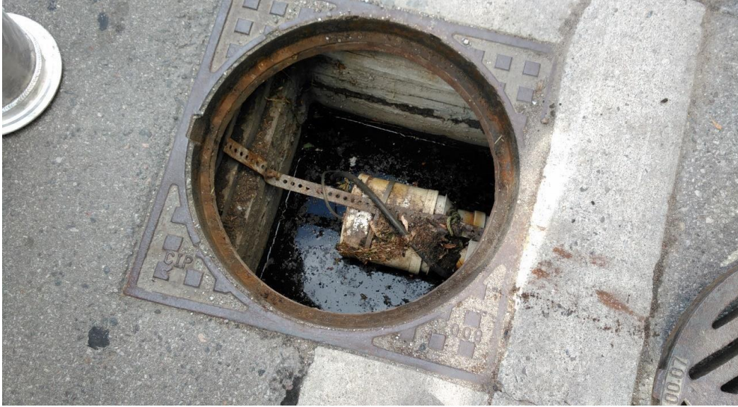
Figure 15. Inlet Pipe in the Drainage Basin
