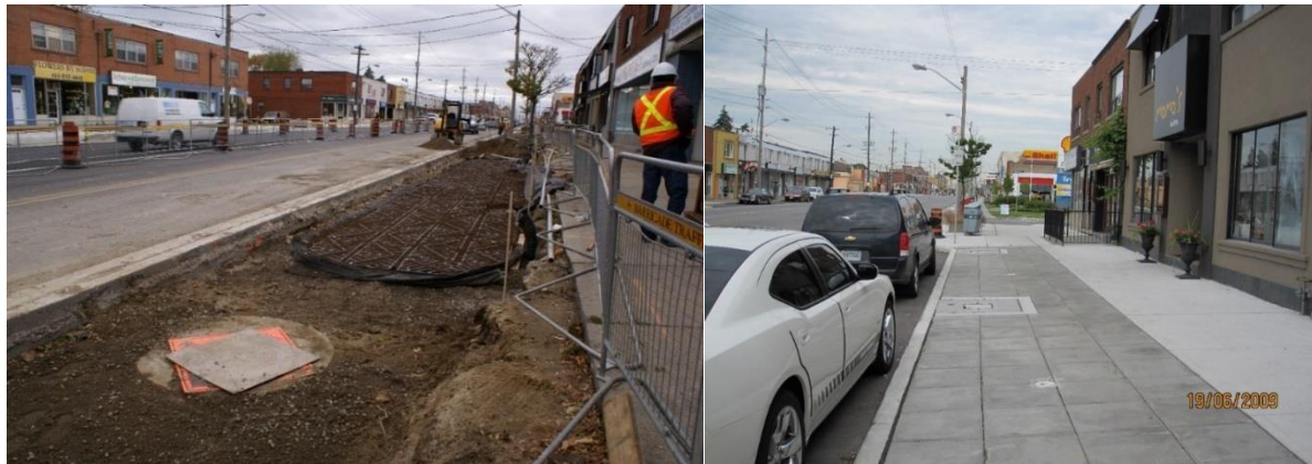
Figure 17. Completed Soil Cell
