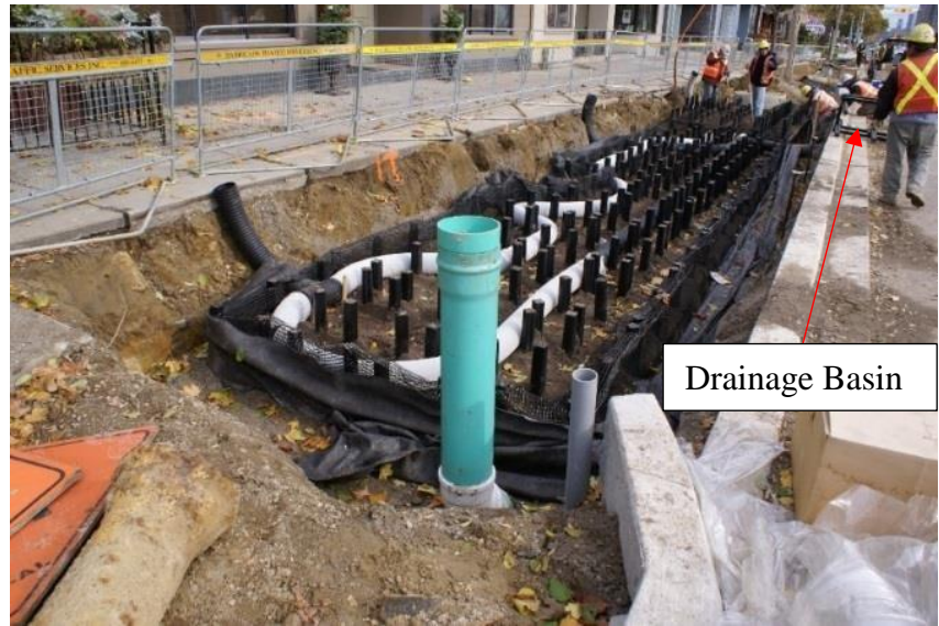
Figure 16. Soil Cell During Construction
