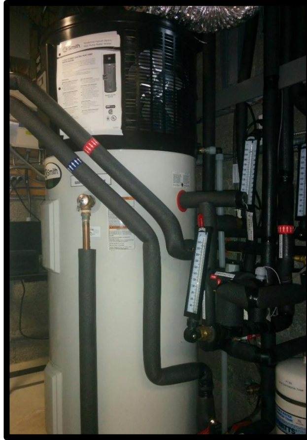
Figure 1-3: Installed A.O. Smith ASHPWH at Archetype House B
