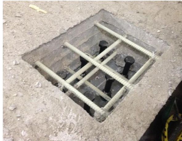
Figure 5.14 Panel-to-girder connection in the transverse direction
