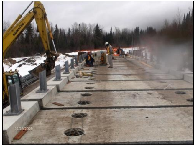
b) Photo of assembled transverse precast deck panels in Passe-à-Fontaine Bridge (source: Hossain and Lam, 2006)
