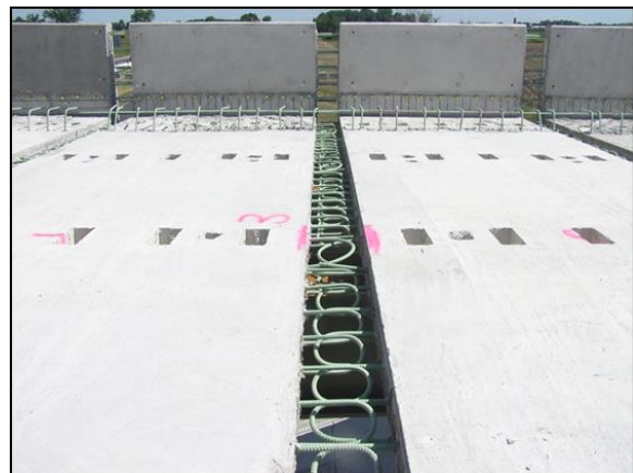
d) Transverse closure Strip in deck and barrier in Hwy 401/Mull Road Underpass (source: Hossain and Lam, 2006)
