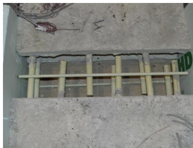
a) Closure strip for slab S3
