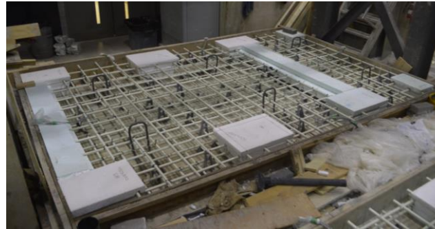
c) View of GRPP reinforcement and and styrofoam to form the joints
