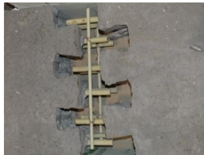
b) Closure strip for slab J.Z.E
