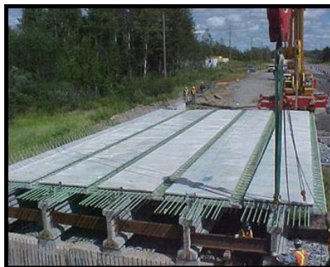
c) Photo of precast girders assembled
