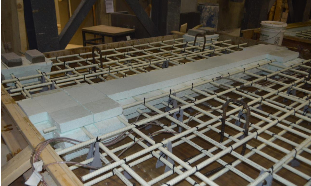
Figure 5.28 Close-up view of forming the C-joint using styrofoam
