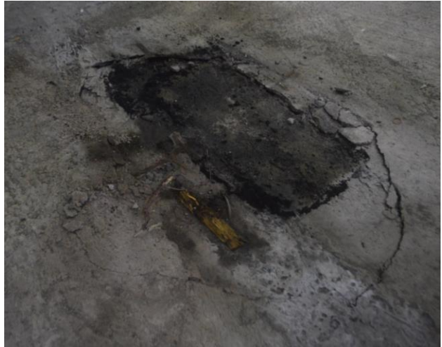
b) Close-up top view for the punching shear failure at the wheel footprint
