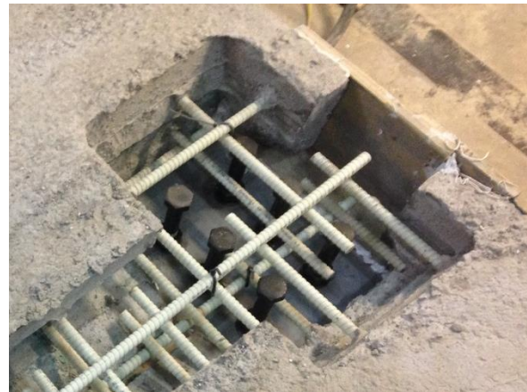
Figure 5.15 Panel-to-girder connection in the longitudinal direction at the edges of the precast FDDP
