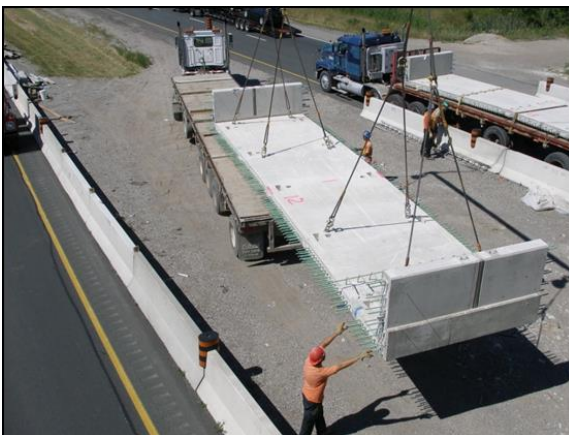
c) Panels off-loaded in Hwy 401/Mull Road Underpass (source: Hossain and Lam, 2006)
