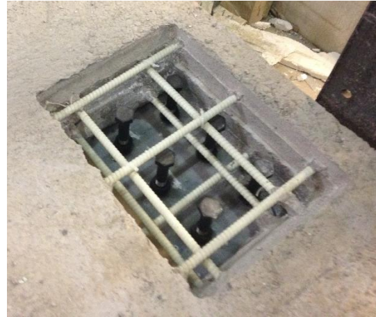
Figure 5.16 Panel-to-girder connection in the longitudinal direction at the mid-width of the precast FDDP
