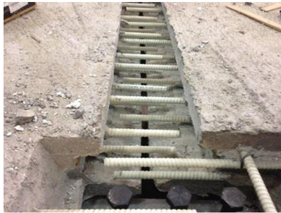
c) Photo of A-joint before adding transverse bars
