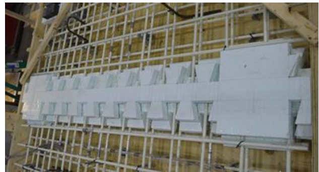
c) Close-up view of the styrofoam forming the joint
