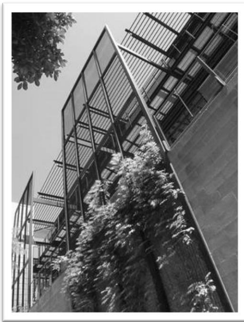
Figure 3 Indirect Green Façade system by Greenscreen®
