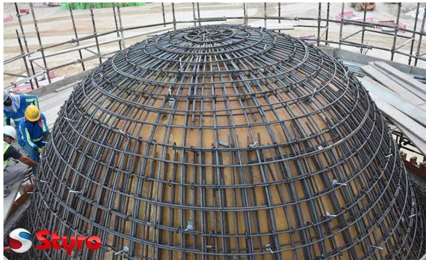
Figure 20. Spherical shell reinforcement (Adapted from https://www.styrouae.com )
