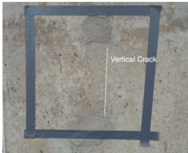
Figure 4.20 - Pier 5-3 Scan Outline and Presence of a Vertical Crack on the Scan Face
