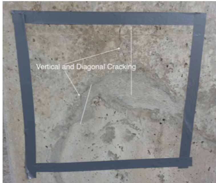
Figure 4.30 - Pier 7-2 Scan Outline with Vertical and Diagonal Cracks Present on the Scan Face
