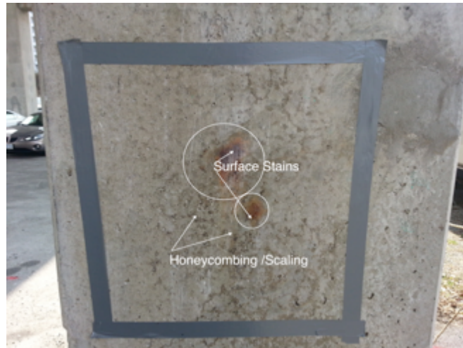
Figure 4.28 – Pier 7-1 Scan Outline with Surface Stains, Honeycombing and Scaling Present
