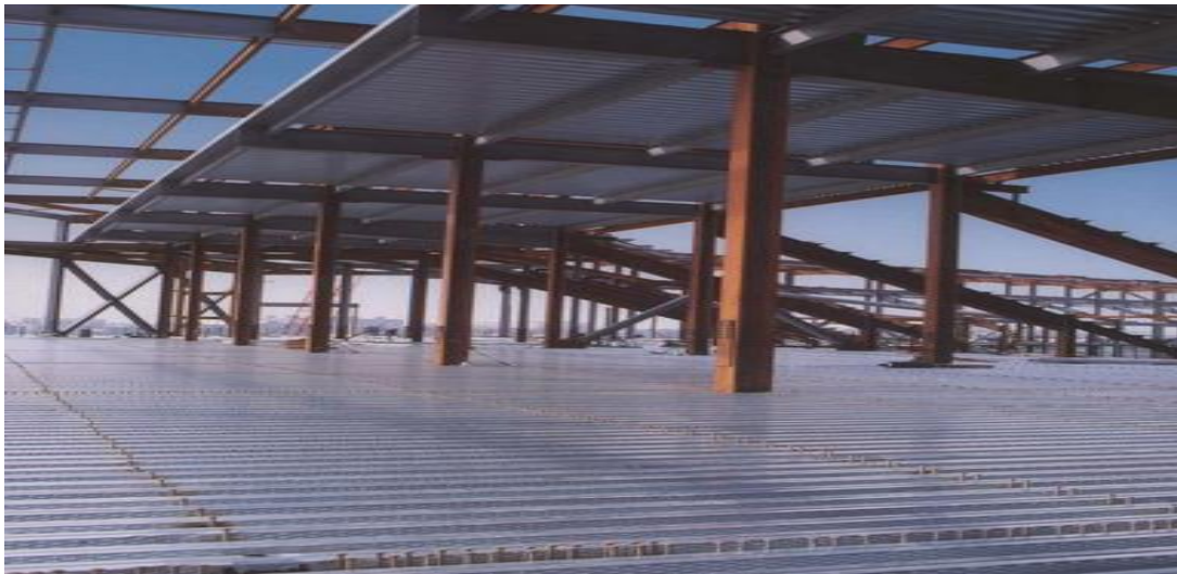
Fig. 2.3:- Typical example of composite slab construction, showing the steel sheet placed on steel frame (Canam, 2014)
