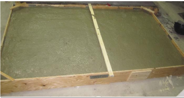
Composite slab after pouring concrete
