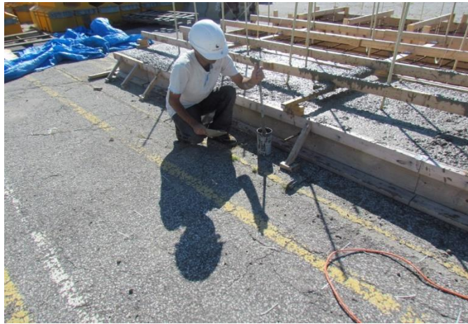
Figure 3. 15 View of taking concrete cylinder specimens from compressive strength test
