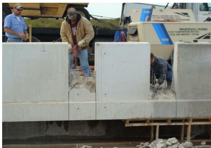
Figure 5. 35 Barrier and reinforcement removal over 500-mm on each side of test barrier
