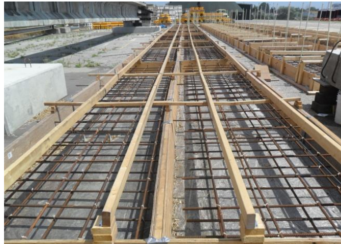
Figure 3. 5 View of formwork of slab models 1 and 2 prior to installation of GFRP bars
