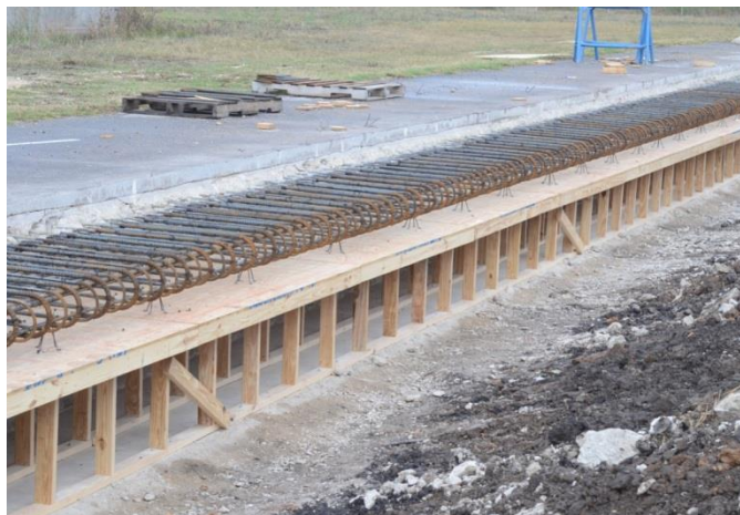
Figure 5. 12 View of steel reinforcement in the deck slab
