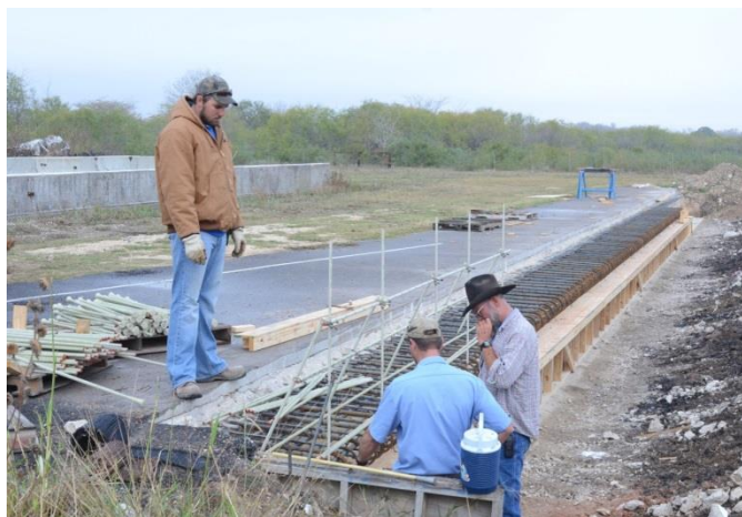
Figure 5. 13 View of GFRP bars installation
