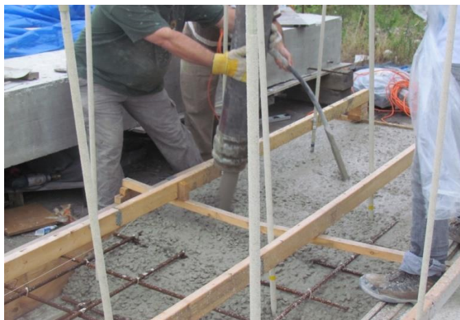
Figure 3. 13 View of concrete casting of slab Model 2
