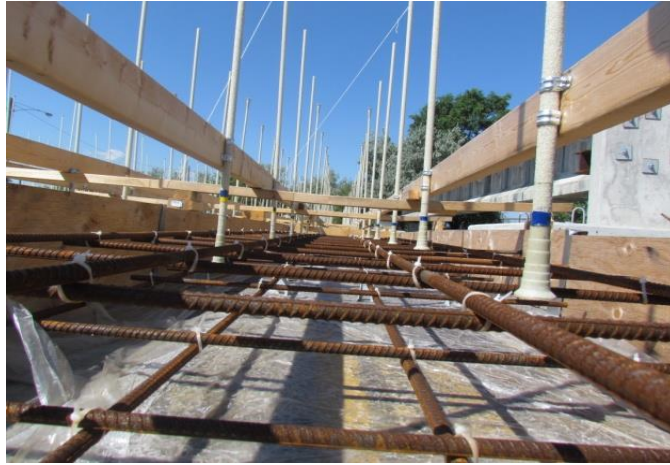
Figure 3. 7 Installation of GFRP headed-end bars in the formwork
