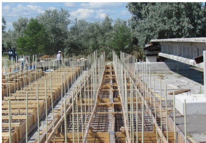
Figure 3. 9 View of GFRP bars in the formwork prior to concrete casting
