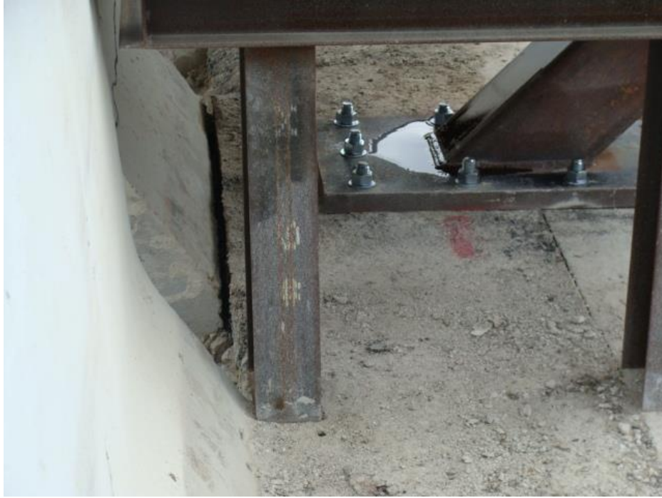
(c) Flexural crack at deck-wall junction
