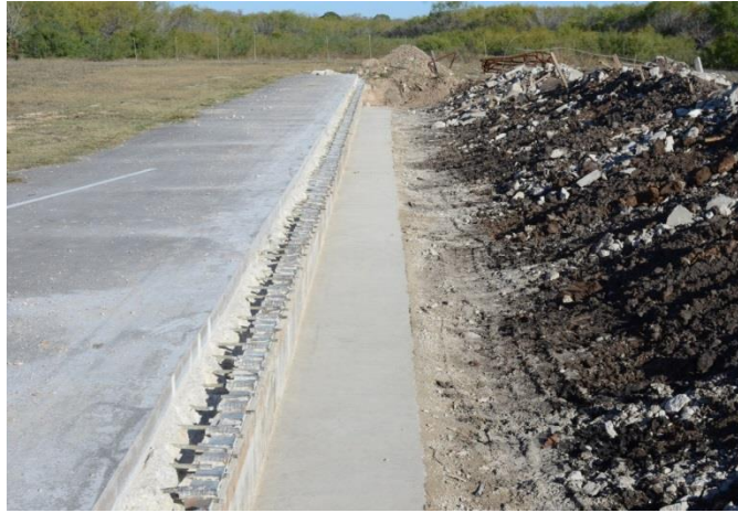
Figure 5. 11 View of the existing concrete foundation with projecting steel dowels at deck level
