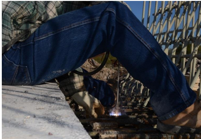
Figure 5. 15 View of welding reinforcing steel in the deck to the longitudinal steel strap
