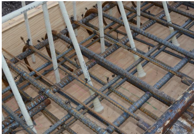
Figure 5. 16 Close-up view of barrier anchorage to deck slab
