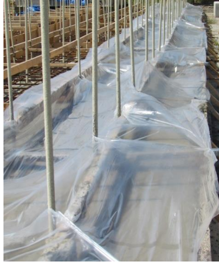
Figure 3. 17 Concrete curing using plastic sheets
