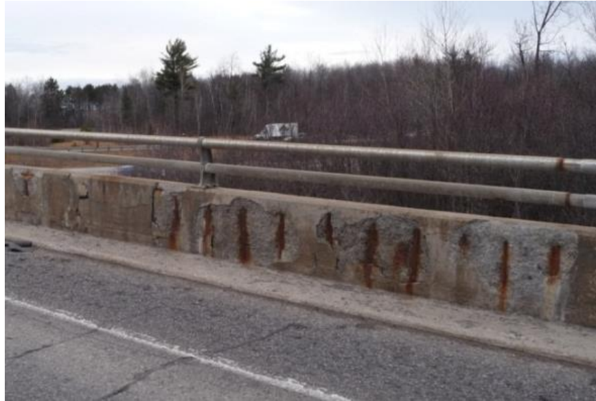
Figure 4. 1 Corrosion-induced degradation of steel-reinforced bridge barrier wall
