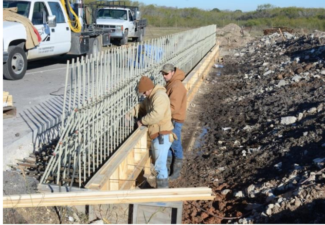
Figure 5. 14 View of the GFRP reinforcement
