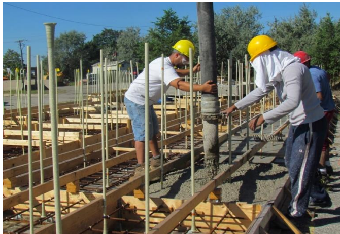
Figure 3. 12 View of concrete casting of slab Model 1
