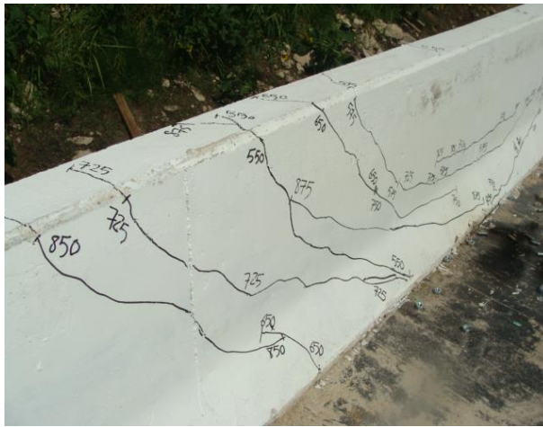
(c) Cracks extending to top of wall thickness
