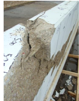
d) Exposed GFRP bars at through crack
