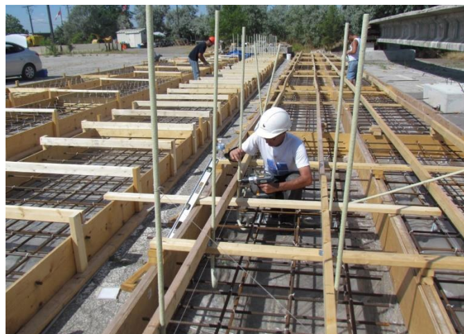
Figure 3. 6 Placement of GFRP hook bars in the formwork
