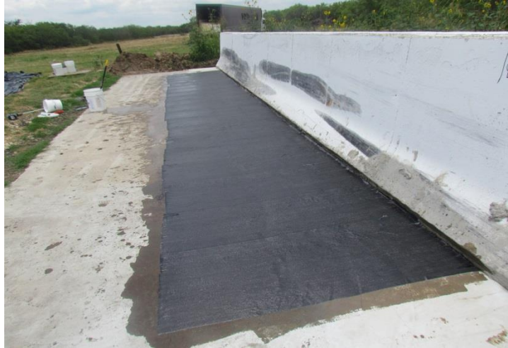
Figure 2. 3 View of concrete slab strengthened with CFRP sheets
