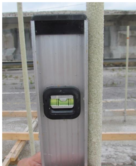
Figure 3. 16 Leveling out GFRP bars after concrete casting to make them vertical in the slab
