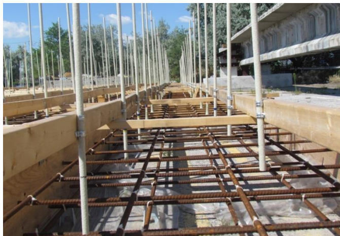
Figure 3. 8 Placement of GFRP straight-end bars in the formwork
