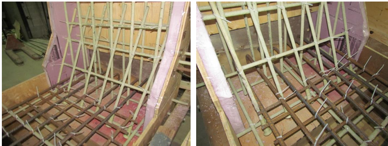
Figure 4. 8 Views of GFRP bars in barrier Model 4
