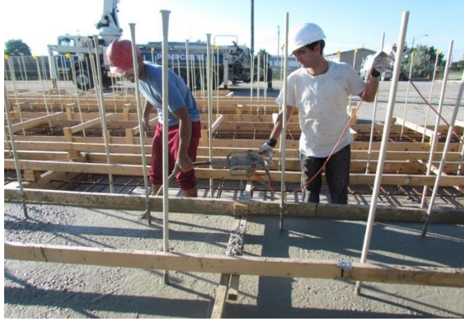
Figure 3. 14 Vibrating concrete during casting to remove entrapped-air
