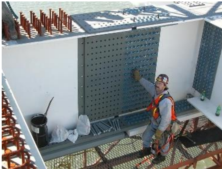
Figure 2-21: Worker installing bolted slip-critical joint on bridge girder (Sternier, 2005)
