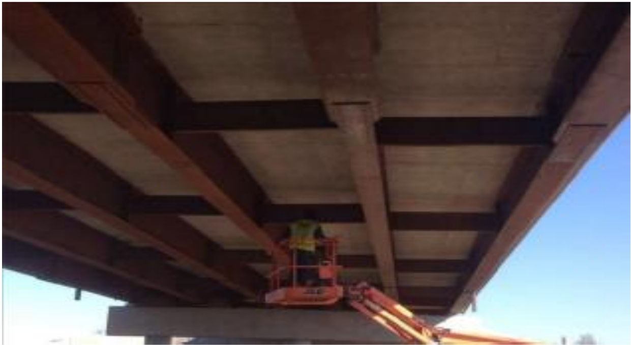
Figure 2-7: Iowa bridge showing the 2 A1010 girders on the far right (Iowa DOT, 2016)
