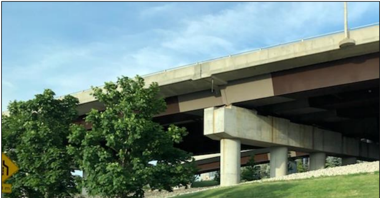
Figure 1-2: Weathering steel girder coated 3 meters apart from the expansion joint
