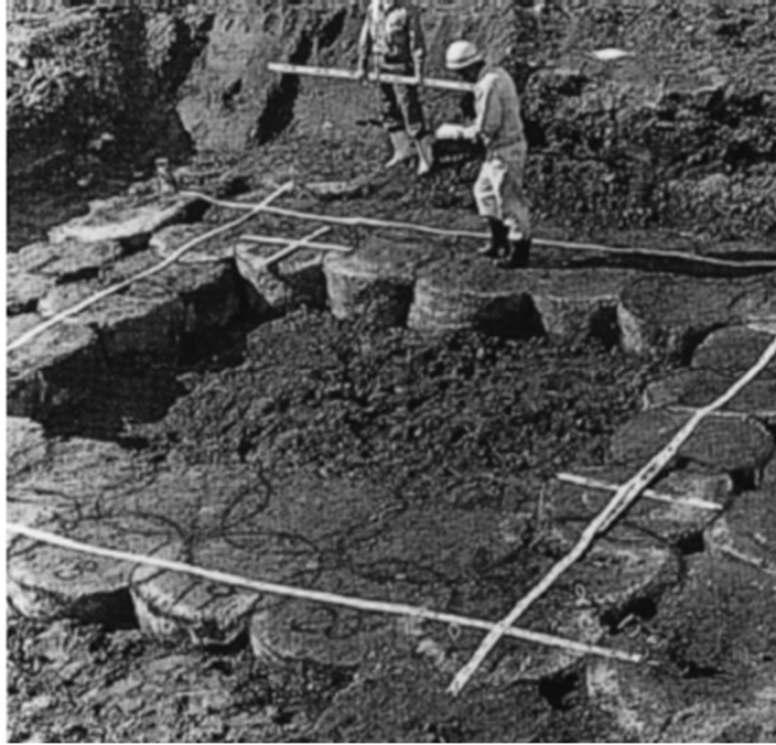
Figure 2-9: Lattice Arrangement of DSM Columns for the Purpose of Liquefaction Mitigation (Porbaha et al., 1999)
