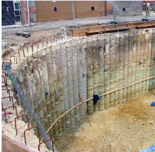
Figure 2-8: A DSM Retaining Wall (Denies & Huybrechts, 2017)
