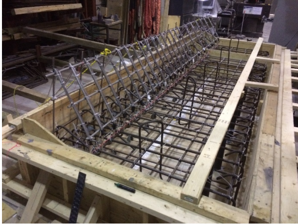
a) Reinforcement before casting the base
