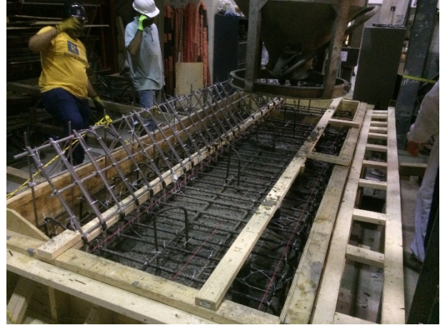
b) Reinforcement during casting the base
