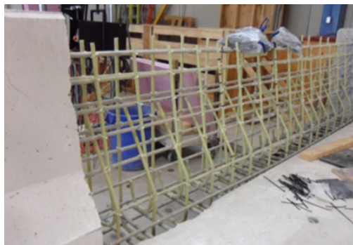
Figure 2.16 Planting method used to replace GFRP at interior location of barrier (El-Salakawy & Rubiat Islam, 2014)
