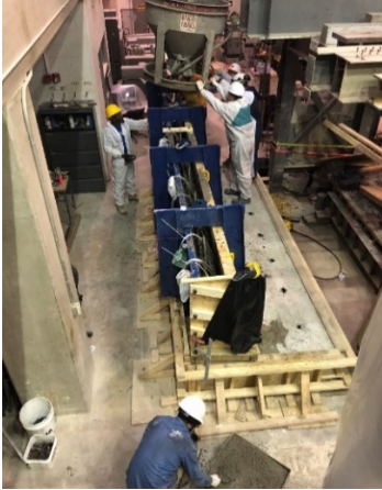
g) Casting the barrier wall
