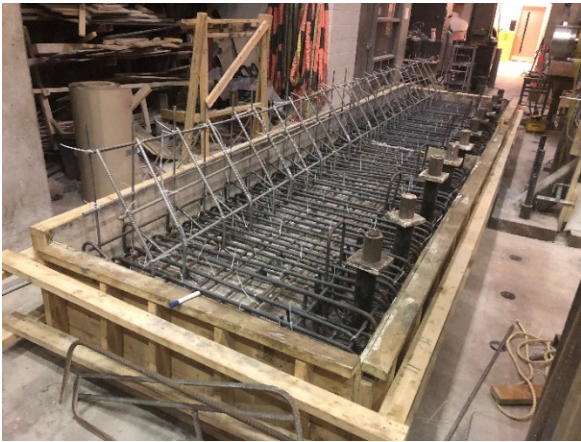
a) Reinforcement before casting the base
