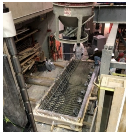
b) Casting of concrete base
